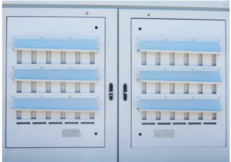
We've installed rain guards on the inverters to protect electrical equipment from water damage.
